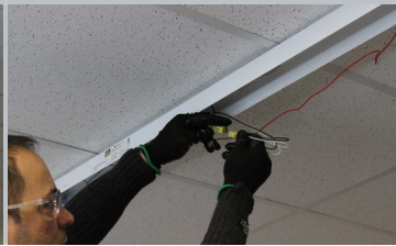
Step Three: Disconnect Ballast from incoming feed. Remove ballast along with socket straps (saddles), sockets and any other lamp retaining clips/hardware. (Recycle/Discard)
