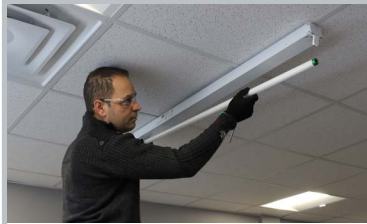
Step One: Remove lamp(s) and set aside for proper Recycling
