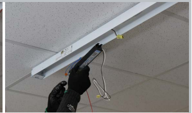
Step Three: Disconnect Ballast from incoming feed. Remove ballast along with socket straps (saddles), sockets and any other lamp retaining clips/hardware. (Recycle/Discard)
