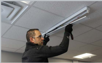
Step Two: Remove Ballast Cover and Recycle/Discard
