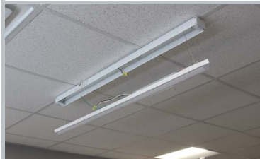
Step Four: Using tether cable (supplied), hang Retrofit tray from an existing hole in housing to be retrofitted as seen above. Connect ground wire from LED Retrofit tray to the fixture housing by connecting to the existing ground wire/ground screw of fixture.
