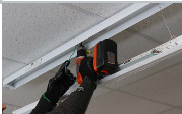
Step Four: Using tether cable (supplied), hang Retrofit tray from an existing hole in housing to be retrofitted as seen above. Connect ground wire from LED Retrofit tray to the fixture housing by connecting to the existing ground wire/ground screw of fixture.
