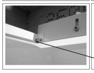
4. INSTALL END SPACER BARS AND TIGHTEN SCREWS.
