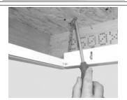
6. INSTALL SAFETY CHAIN (BY OTHERS) FROM HOLES PROVIDED ON THE TOP OF SIDE FLANGE ASSEMBLY TO THE CEILING STRUCTURE.
